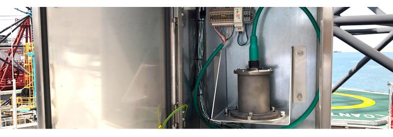
To extend the motion sensor lifetime SMC recommend using a protective enclosure during offshore installations. The optional enclosure provides additional protection to the motion sensor when required.
